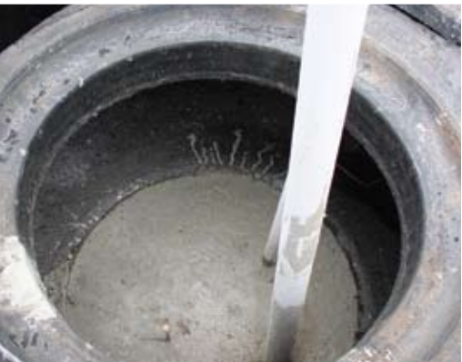
Fill the bottom center bead area of tires with concrete, and tamp it to seal tight around the edges.
